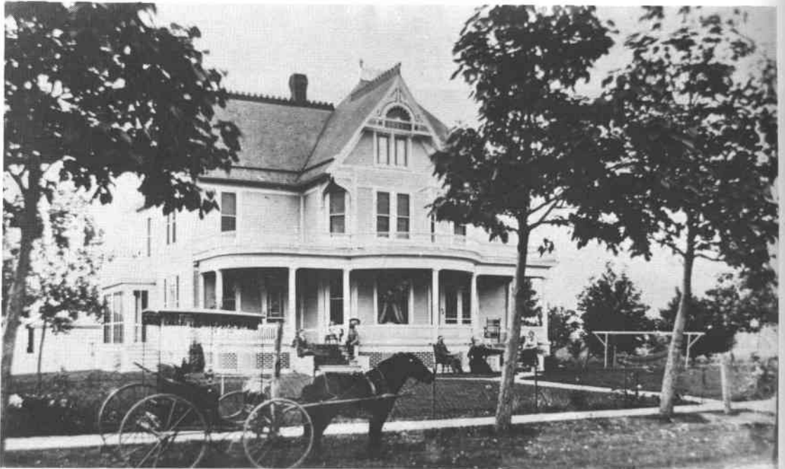
A marvelous porch, which extended across the entire front of the house, and which could accommodate the entire family, plus visitors. Note the low fence between sidewalk and yard.
